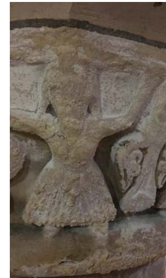
Stone corrosion
