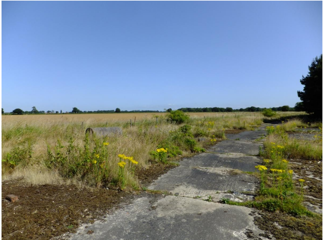
Plate 12 Part of perimeter road around N end of runway complex, looking NE
