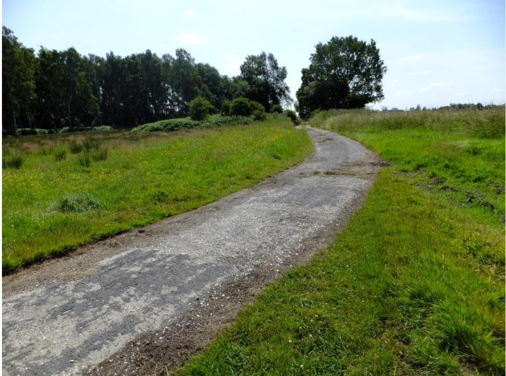
Plate 13 Part of RAF perimeter road to NW side of Moor Plantation, looking S
