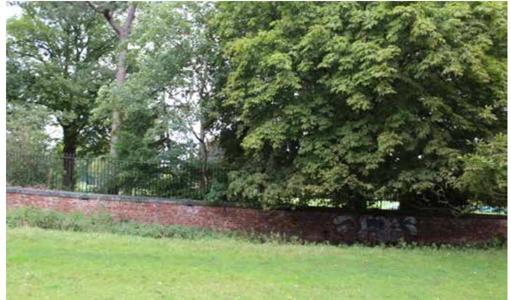
▲ E. The high brick wall along the western edge reduces in height and is replaced with railings for a portion of the boundary before returning to a high wall.
