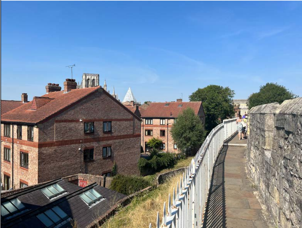
PLATE 7: Foss Bank - Monk Bar View north-west. 3-storey modern housing to the west, left of image, part of estate development around Aldwark.
