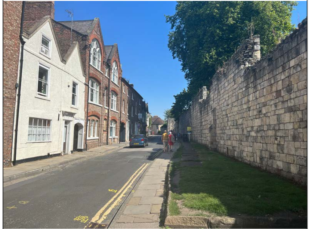
PLATE 10: Marygate - St. Mary's Abbey Walls View north-east from along Marygate.
