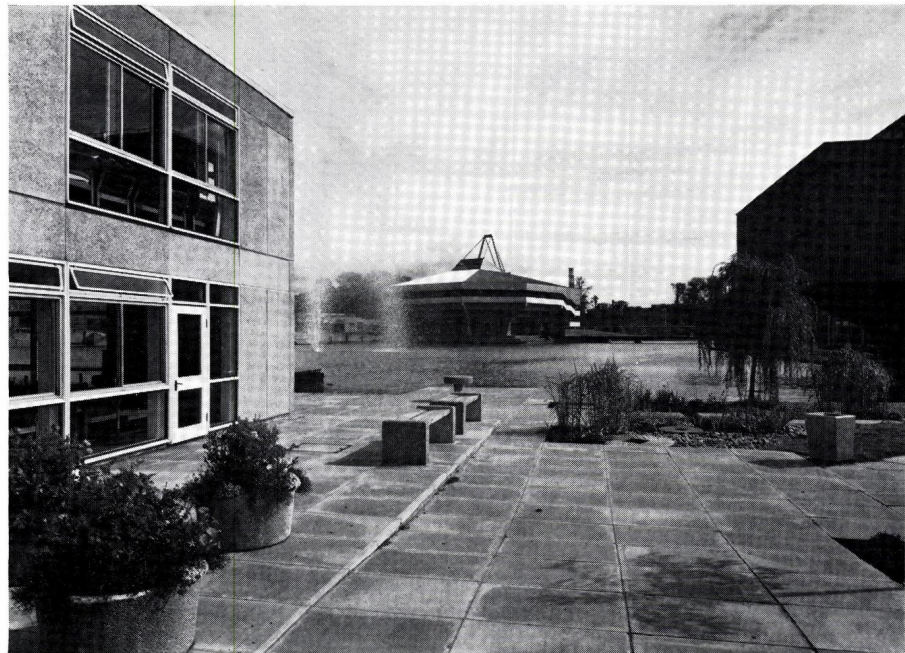
5.—THE HARBOUR-LIKE BASIN AROUND THE CENTRAL HALL OF THE UNIVERSITY. The large paved areas have been designed to provide constant variation in level, material and style, which are further diversified by low-growing plants
