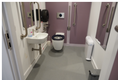
The accessible WC on floor 2a which measures 1430 mm wide x 1880 mm deep.
