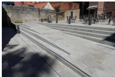
The steps and ramp within the Yard and uneven height risers.
