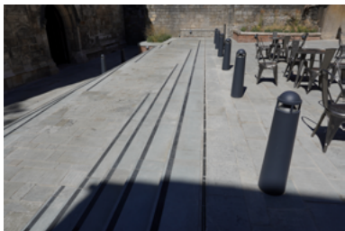
Bollards with lighting included.
