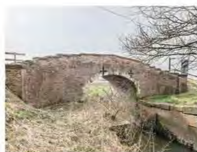
Strensall New Bridge - Haxby Moor Road
