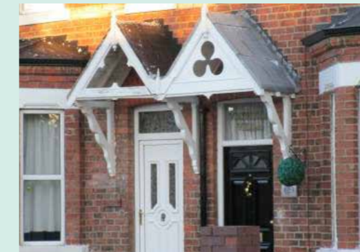
Photo 45: View of decorative detailing
