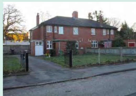
Photo 16: Housing on south side of Alexandra Road
