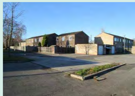
Photo 19: Housing to the north of Howard Road
