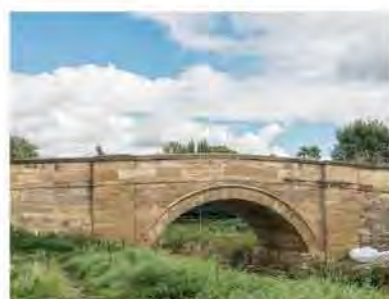
Strensall Bridge - Sheriff Hutton Road
