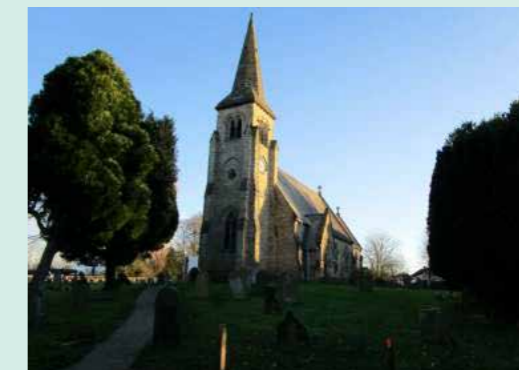
Photo 8: View of St Mary's Church
