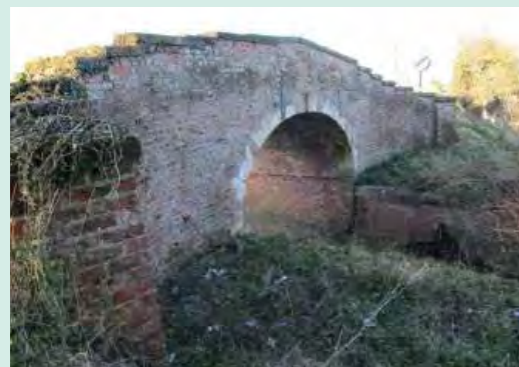
Photo 9: Strensall New Bridge
