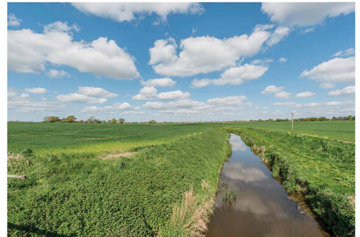
a2. Northeast from Towthorpe Bridge
