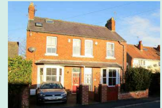
Photo 24: Example of nineteenth century semi-detached housing
