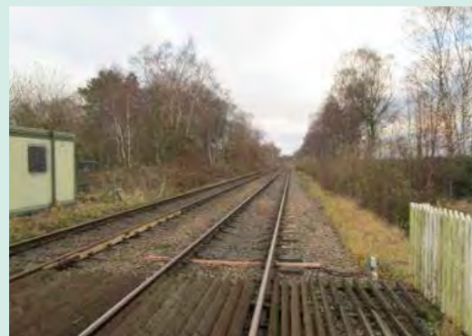
Photo 3: View of the railway line
