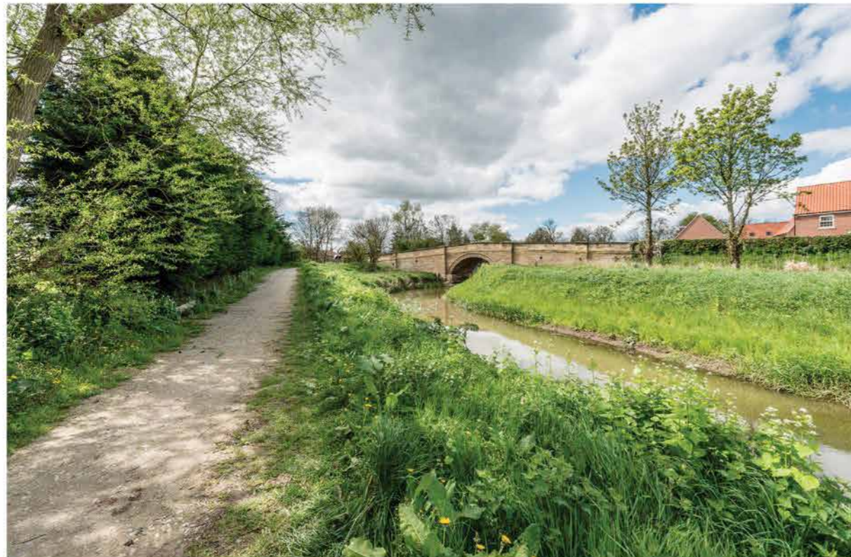
c1. South West towards Strensall Bridge (John Carr's Bridge) from the Foss. The views of the bridges from the riverside pathways are valued locally. Villagers recognise the importance of retaining pathways along the length of the River Foss through the Village
