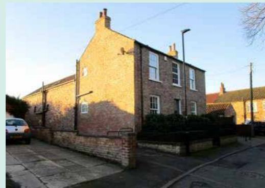
Photo 34: Example of detached house with rear wing
