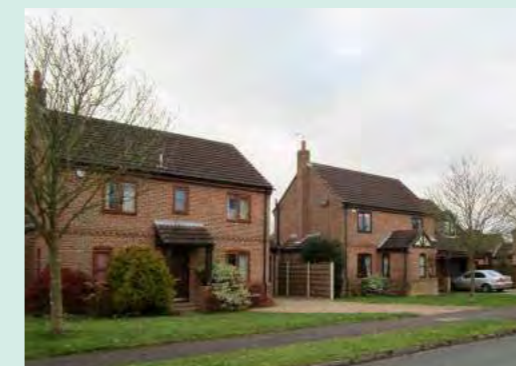
Photo 25: Twentieth century two storey housing
