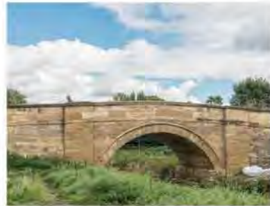
Strensall Bridge – Sheriff Hutton Road
