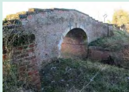
Photo 9: Strensall New Bridge
