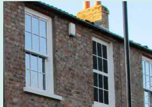
Photo 40: Example of a red clamp brick
