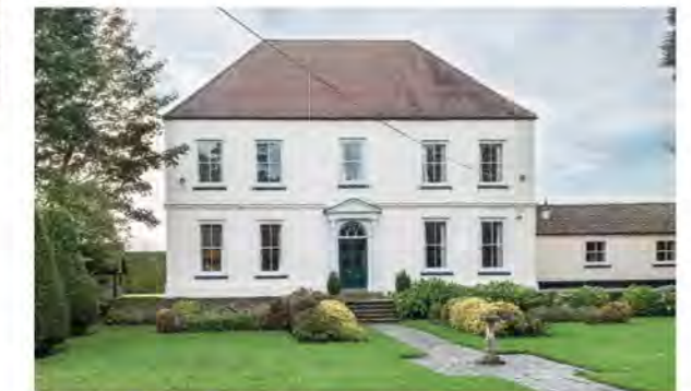
Manor House Farmhouse, Strensall
