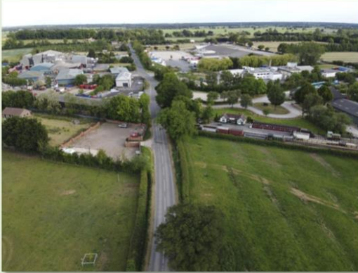
The industrial estate on Murton Lane. The farm leading to the boundary is devoted to livestock. In the foreground on the right of the road is Murton Park Station of the Derwent Valley Light Railway and Murton Park which contains the Yorkshire Farming Museum. Beyond them are the ABP Food Group abattoir and the York Auction Centre. The buildings on the left include William Thomson (York) grain depot and L Clancey and Sons recycling centre.
