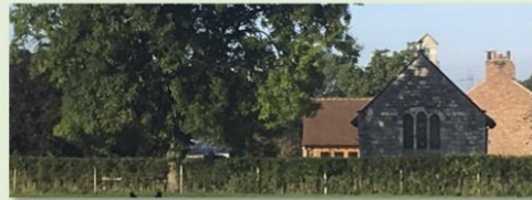
The new Welcome lobby to St James's Church, funded mainly through efforts of the village to enable the church to be used for the whole community
